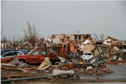
Figure 6: Tornado damage in Joplin, Missouri, May 23, 2011, KOMUnews, Creative Commons.
